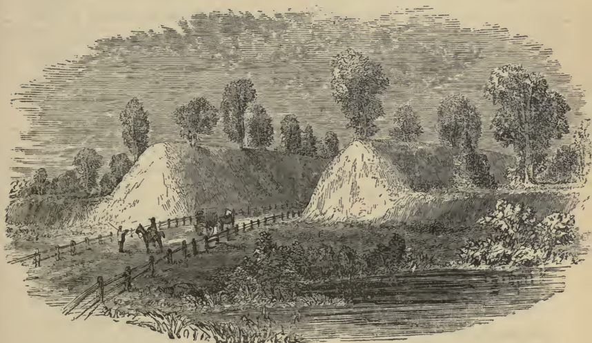
GRADED WAY NEAR PIKETON, OHIO.
